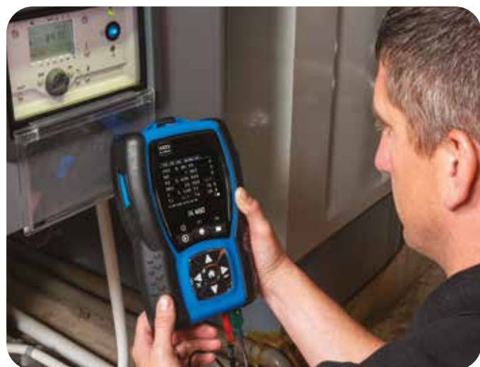
Confirm boiler safety & efficiency
