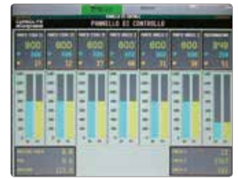
Display showing control zone temperature and setpoint, % power, lance thermocouples, height indicator and wall pressure.
